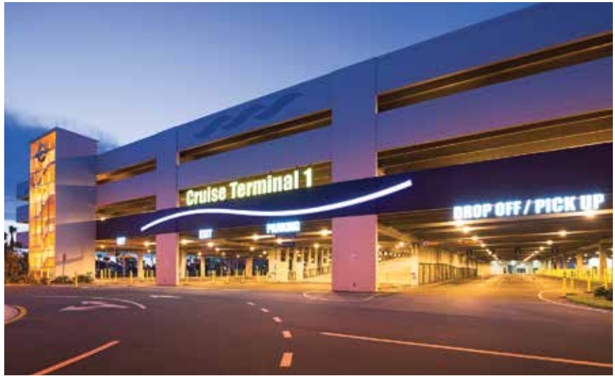
Cruise Terminal, which was recently completed, features passenger drop-off and baggage-handling services on the first level, with parking spaces on the second floor up. The 433,764-square-foot project was constructed, along with the new terminal, in less than 12 months to serve the Royal Caribbean line. Photo: Finrock.
