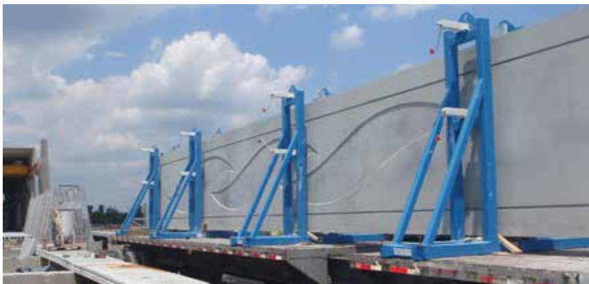
Spandrels with the port's logo cast into them are shown. Two crews were used to shorten the schedule and keep it off the critical path of construction for the terminal being built. Photo: Canaveral Port Authority.
