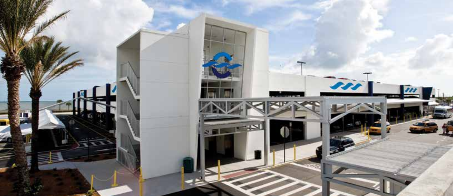
Precast concrete spandrels had the terminal's blue logo cast into them, after which they were painted to create a dimensional appearance. Photo: Finfrock.
